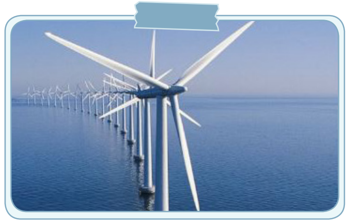
Picture 6. Working Wind Turbine
